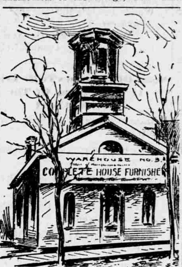
OLD CHURCH, NOW A WAREHOUSE.
