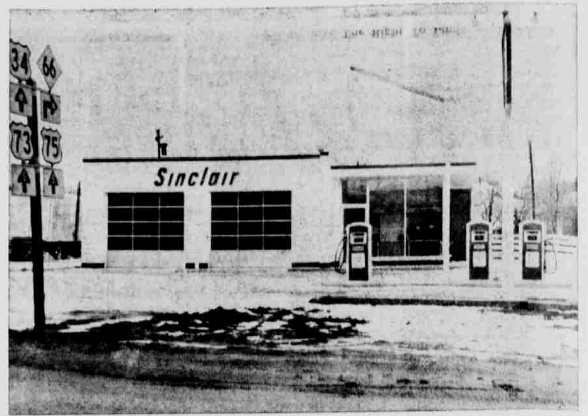
NEW BUSINESS—This new Sinclair Service Station will begin operating Tuesday at Chicago Avenue and Hill Street. Proprietors are Les Hutchinson, bulk man, and Joe Gochenour, service station operator. The station was constructed by Young and Jose Building Contractors.
