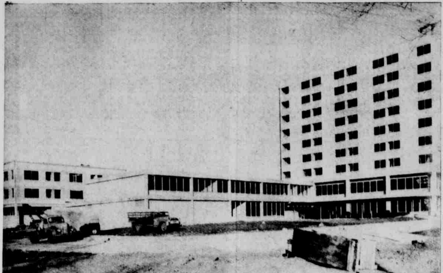
NEBRASKA CENTER FOR CONTINUING EDUCATION—Workmen soon will be putting the finishing touches on the Nebraska Center for Continuing Education which opens June 1 on the University of Nebraska College of Agriculture campus. The Nebraska Center, and an integral part of the facility, the Hall of Youth, was planned nearly three years ago when the W. K. Kellogg Foundation of Battle Creek, Mich., contributed $1.5 million and business and personal gifts of Nebraska gave another $1 million for its construction. Some 50 educational conferences, institutes and workshops already have been scheduled to be held in the Nebraska Center. —(College of Agriculture Photo).
