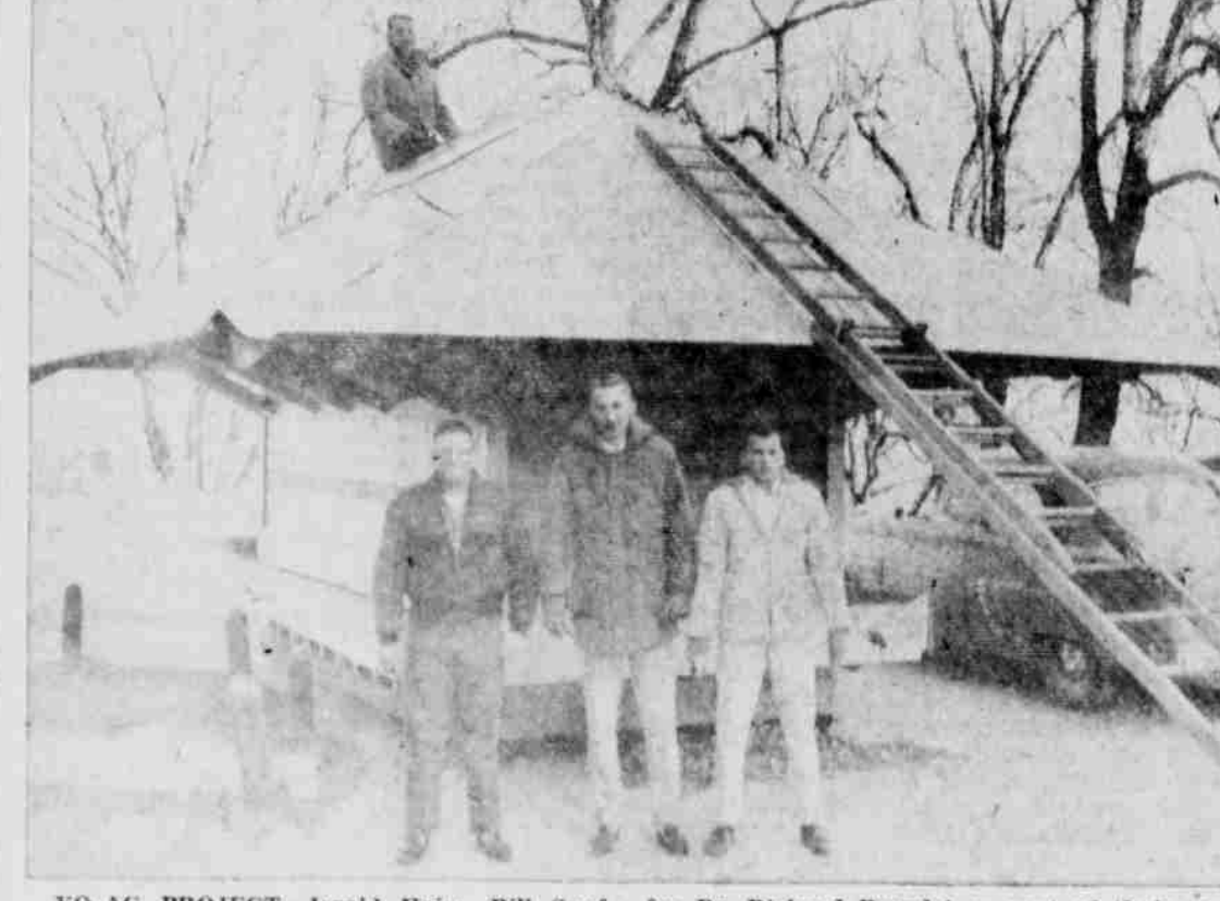
VO-AG PROJECT —Jerald Heim, Bill Senf, Roger Mrasek (left to right on ground) and Ron Tilson (in the loading hatch) are shown with the cattle self-feeder they designed and built for Dr. Richard Brendel as part of their vocational agriculture program at Plattsmouth High School. The feeder will hold 600 bushels of grain.
