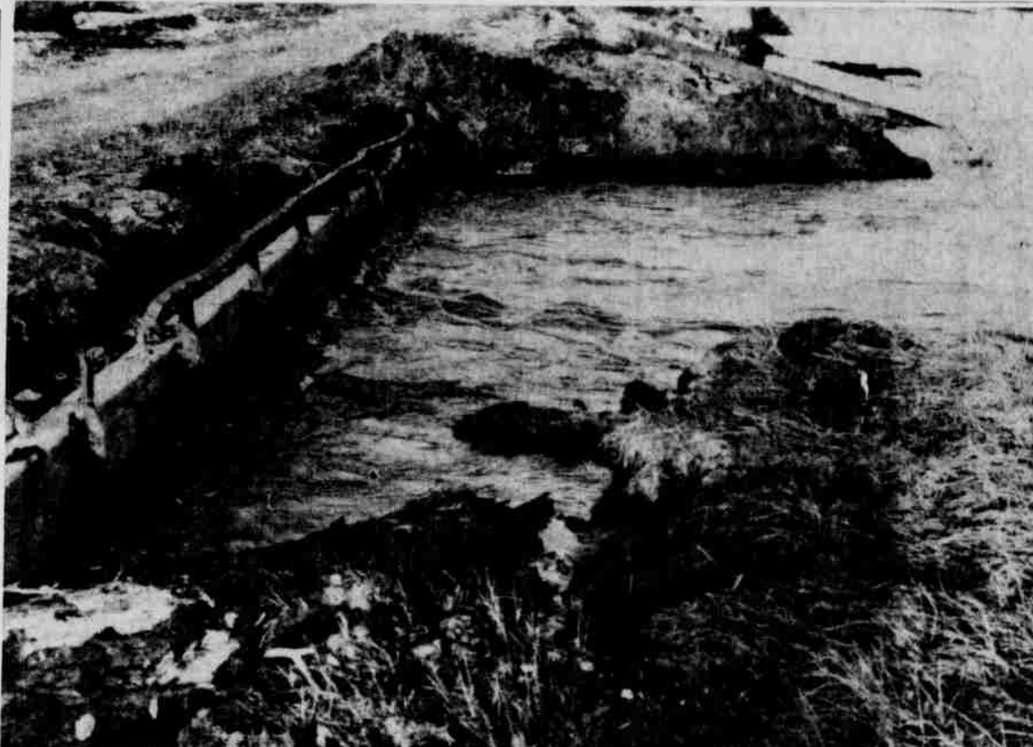
ESCAPE VALVE—This concrete bridge and culvert was the escape outlet for water trapped by the river road in the acreage north of the road. Sunday the culvert, long covered, was opened to get the water draining. Most of the water was gone in a few days but low spots still have accumulations.
