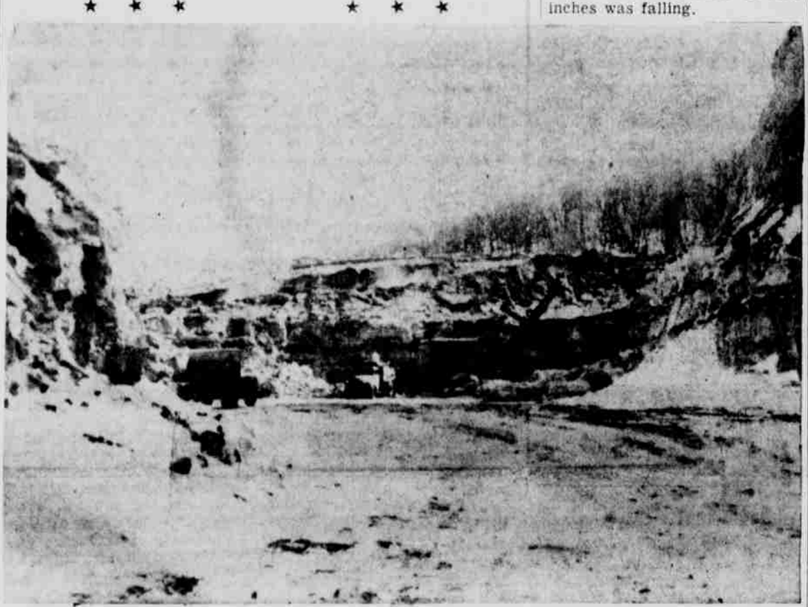
QUARRYING —"Rip-rap" is loaded with a power shovel which was keeping a half-dozen trucks driving hard to keep up. Rock is weighed on a portable scale near the quarrying site. This year, $1,200,000 worth of this kind of dike work is up for contract along the river here and south of here.
