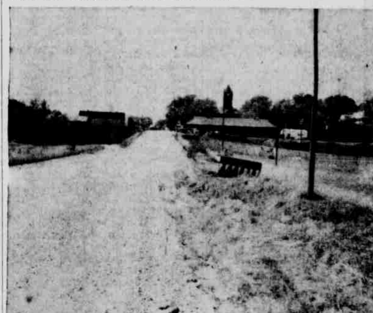
FROM THE EAST , the crossing looks like this. Work was still being done on the grade of the road which intersects the crossing approach. The road will lead north past the city water plant to the Game Commission's Wildlife Management Area (old rifle range).
