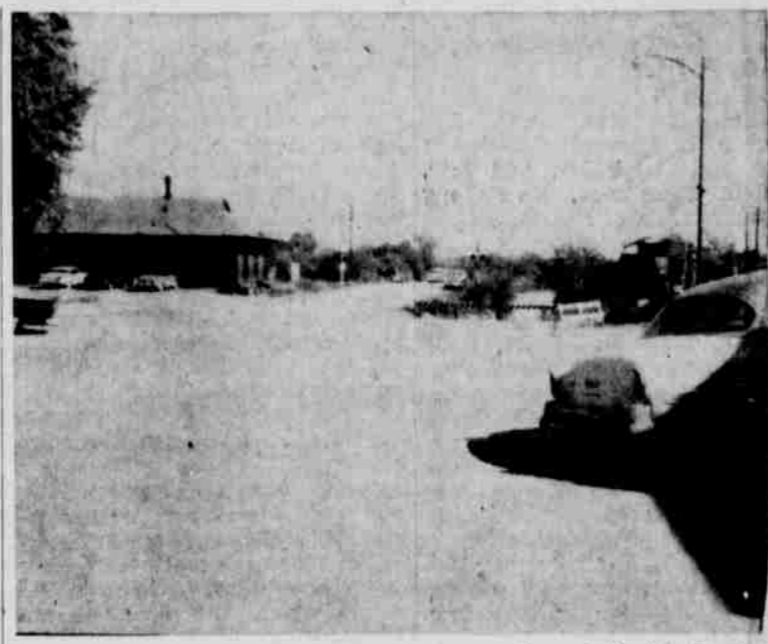
GRADE CROSSING — The grade crossing of the Burlington Railroad tracks here went into operation Friday when the railroad erected a barricade to close the underpass for so many years. The underpass now will be only a drainage outlet. The view above was taken from lower Main Street.
