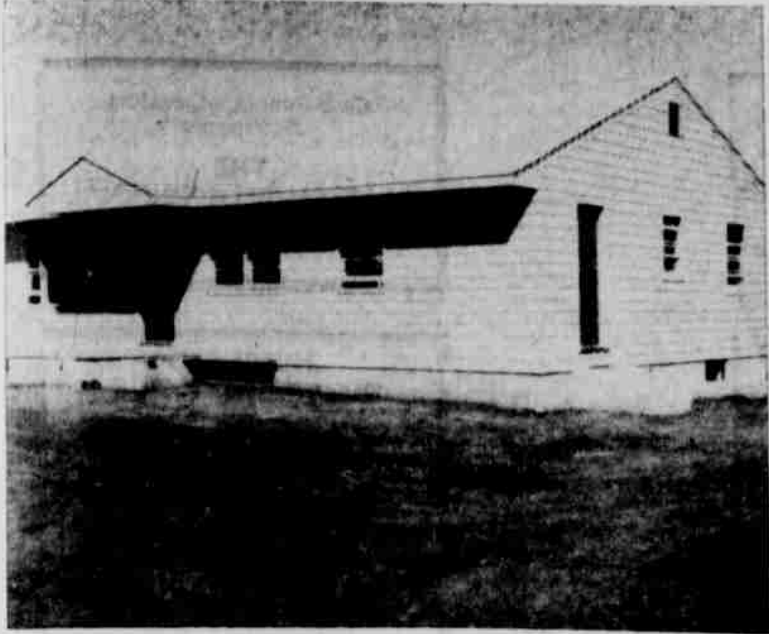
THIS IS THE FIRST house to be erected in the New Ideal Heights situated between Highway 73-75 South and Lincoln Ave. Andrew Epperson of Council Bluffs, Iowa, is developing this area.
