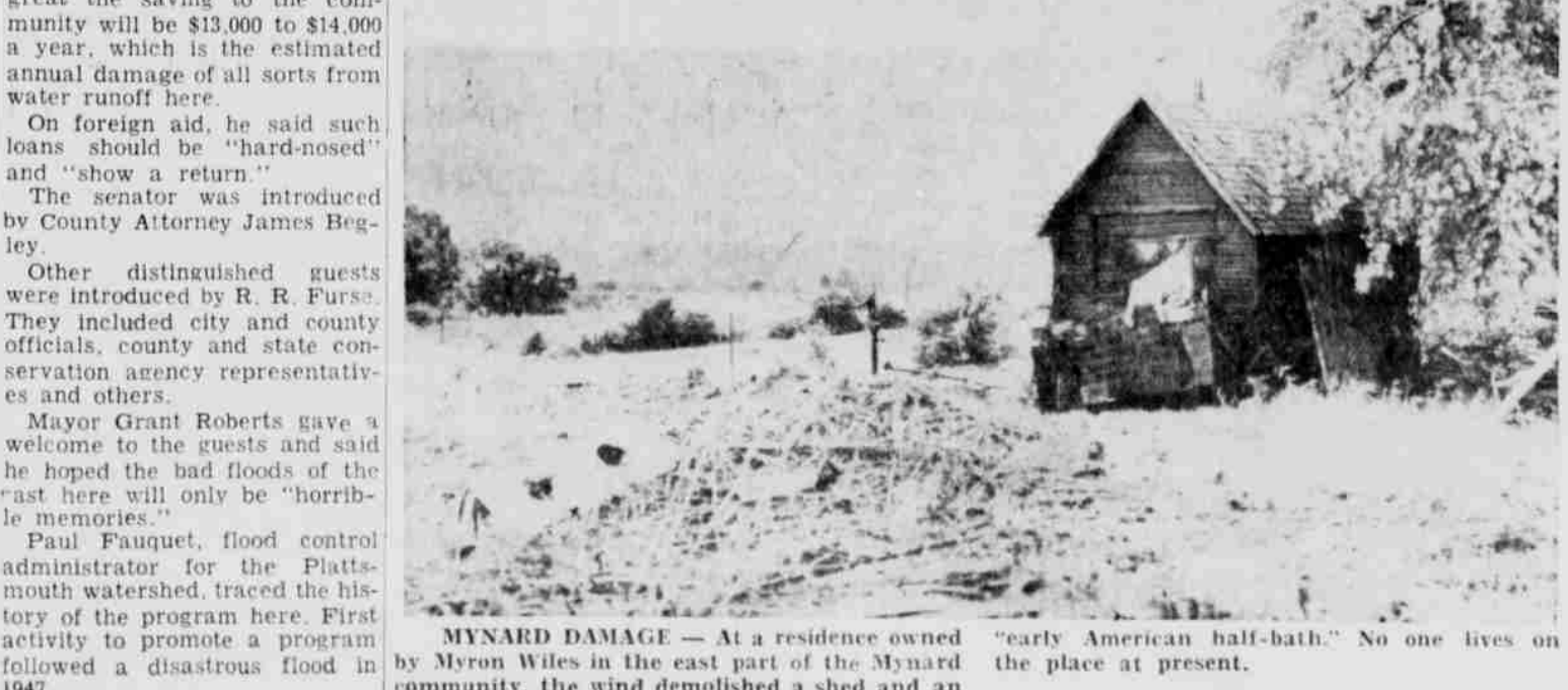
MYNARD DAMAGE — At a residence owned by Myron Wiles in the east part of the Mynard community, the wind demolished a shed and an "early American half-bath." No one lives on the place at present.
