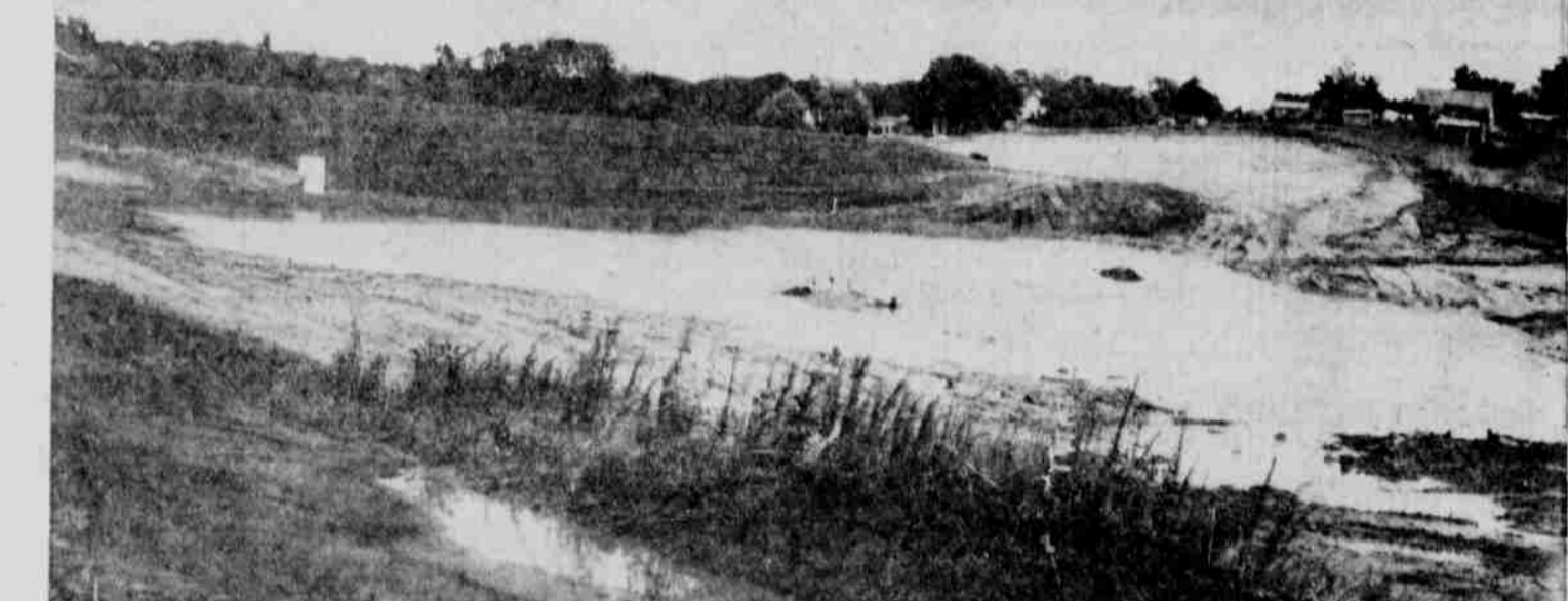
'HILL CITY LAKE' — The new lake behind Dam 10-A was only about two hours old when this photo was taken looking northeast from the Missouri-Pacific RR track. Three boys are near the "island at center". They seemed to enjoy the water although it was thick. There were also two dogs in the muddy drink.
