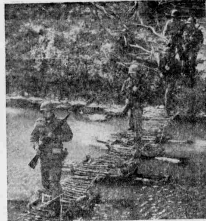
FIELD EXPEDIENT—Shelter halves, carried by every infantryman, available sticks, a half hour's time, and know-how imparted by veteran sergeants resulted in the foot bridge being crossed by these trainees at Fort Hood, Tex. The recruits quickly learn to make do in the absence of engineers.
