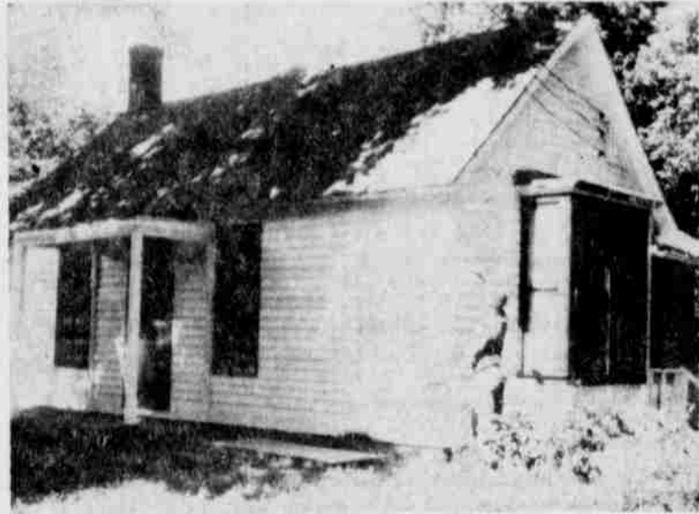
AFTER — Bright and shining as a new penny, the house is pictured Sunday about 4 p.m. as the last of the workers completed the final touch-up. Don Born can be seen at the corner of the house. The Jaycees also trimmed the large tree which had limbs brushing the house.
