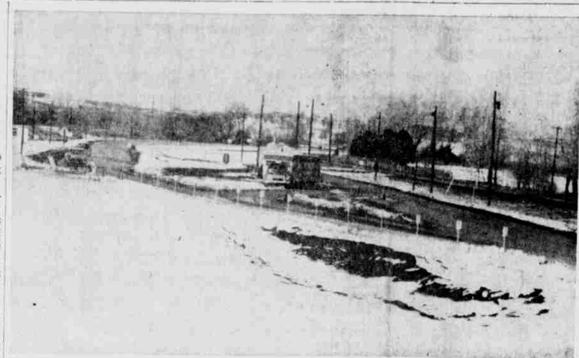
NEW LANE OPEN — The new west lane of U. S. 73-75 to Omaha was opened to traffic Jan. 20 from just south of the Platte River bridge, on north to Omaha. The scene above looks north at the weighing station where single lane traffic now ends for northbound travelers.
