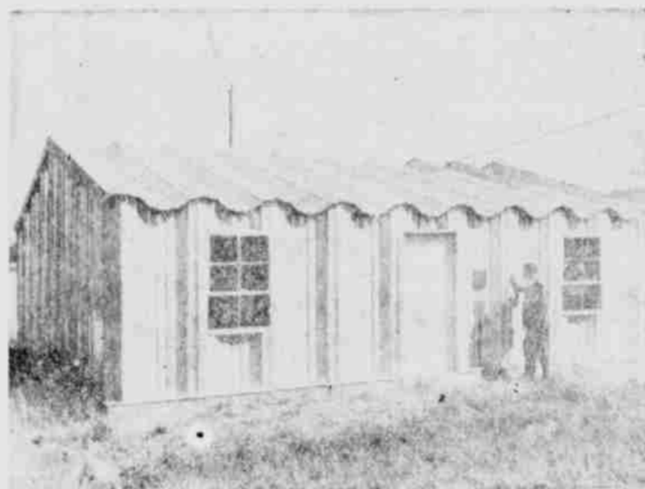
ATOMIC TEST BUILDING — This frameless metal building which faced up to the atomic blast in 1955 at Yucca Flat, Nevada, is being donated to the College of Agriculture at the University of Nebraska by the Behlen Manufacturing Company of Columbus. George Peterson, member of the Department of Agricultural Engineering at the College, reads the plaque stating this building was located 15,000 feet from a nuclear explosion. — (College of Agriculture Photo)
