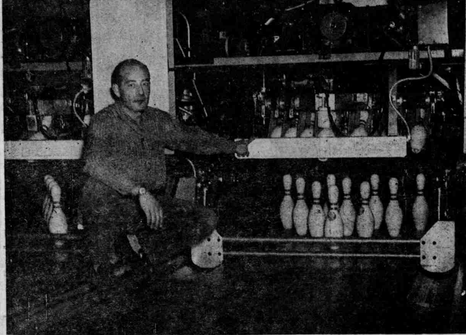
THE LATEST thing in automatic pin setting equipment has been installed and is in operation at the Bowlero, corner fifth and Ave. A. All eight alleys have been installed and is in devices which do away with human pinsetters. In the picture, Howard Hirz is shown pointing at one of the intricate machines. The metal bars stretching across the alley sweep up the pins depositing them on an endless belt at the rear, where they are inserted in the pinsetting machinery. The new equipment will give the Bowlero expanded hours of operation for open bowling on weekends and following league hours during the week. —Journal Photo
