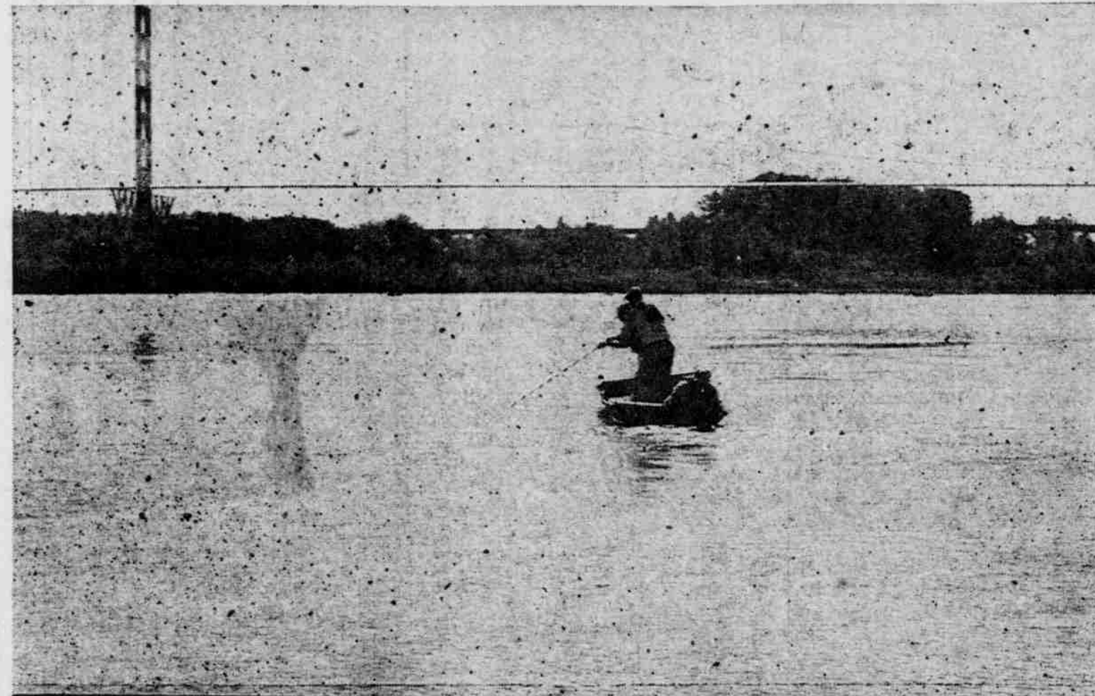
10:15 A. M. — SOLOMON, Hamlin and McGraw start bringing in the line from 40-feet of water near main current of river.
