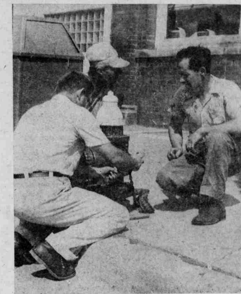
CHANGING HYDRANTS OVER — Fire Chief Joseph Kruntorad is shown looking over the switch of hose connection threads on city fire hydrants. A standard thread was adopted upon the advice of Bruce Wilson, state chief of vacation for fire departments. Others in the picture are Geo. Holman, local fire department truck driver, and Don Wall, a fireman. (Journal Photo).
