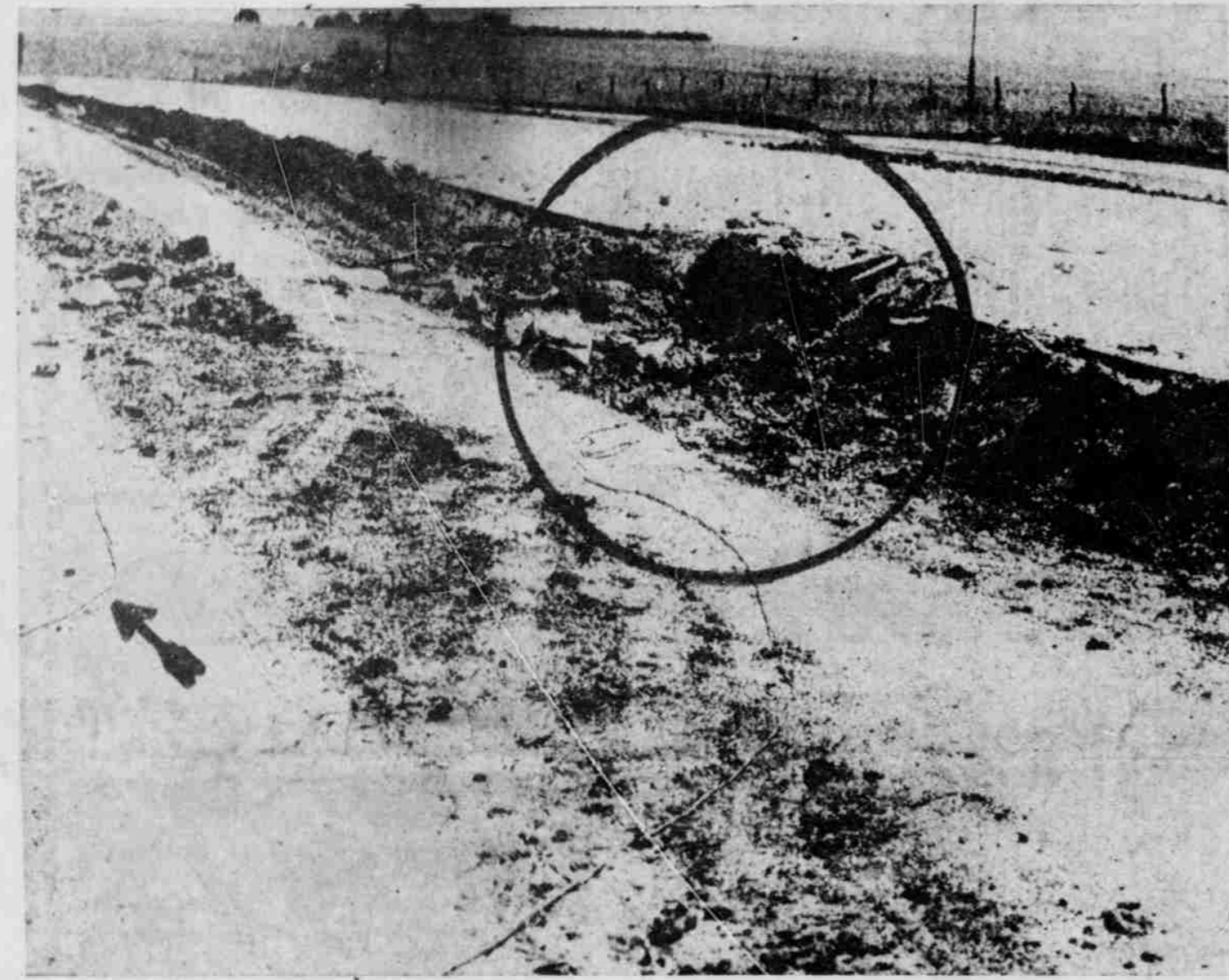
BLOWN UP —Shown above is a portion of new Route 50 blown up by a dynamite blast near Manley. The circle covers the main portion damaged by one of the two separate explosions. Two fuses can be seen running across the roadway. Damage by the blasts is expected to be nearly $1,500. Photo by the Sheriff's Office.
