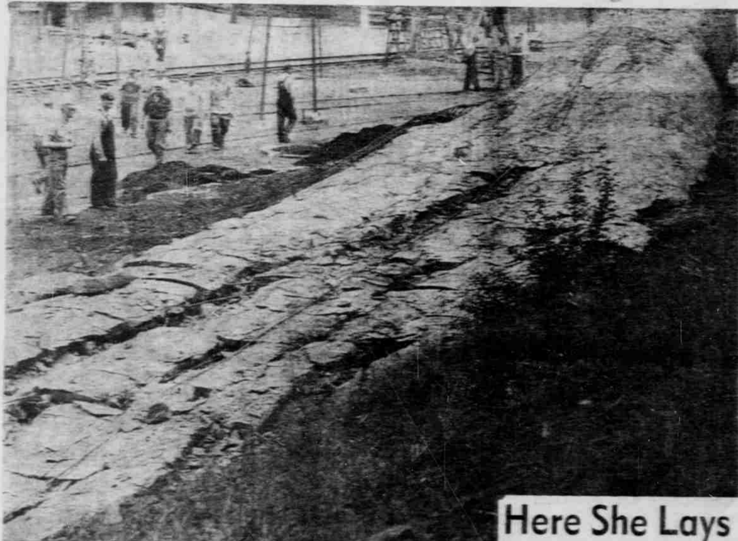
PLATTSMOUTH'S — Tallest structure in shown this past Friday as it fell to the ground after it was purposely undermined by a Chicago demolition crew. The smokestack, highest in the city, crumbled to dust after its fall.
