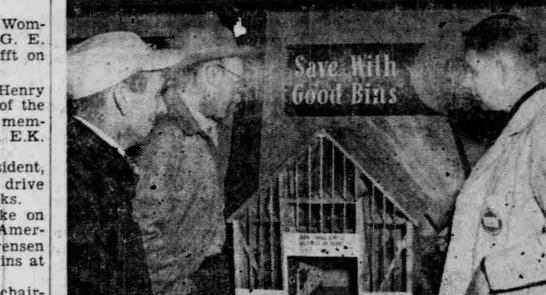
A UNIVERSITY of Nebraska agricultural extension engineer, E. A. Olson, explains some of the more important features of a building designed to dry and store either shelled or ear corn. clothing prices for the months in girls' wear, particularly in The model's exterior, made of clear plastic, enables visitors to see The president, Mrs. E. J. the interior construction of the building. This is one of the ex-Bender, named Mrs. H. C. El- hibits at the 1956 Cornhusker Caravan.
