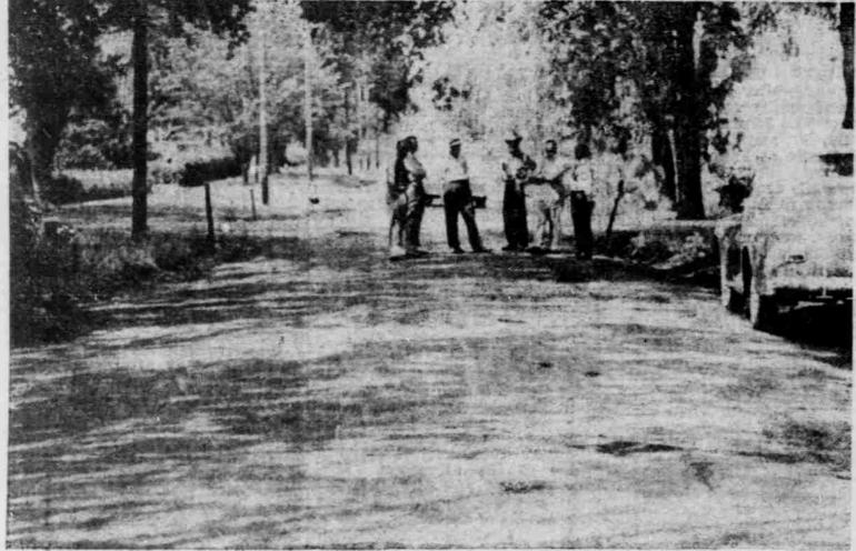
While treatment over gravel or rock is much preferred, the above view of a dirt road in Stanton, Nebr., shows that a dirt roadbed can be made into a permanent all-weather road. There is little difference in appearance, the road is hard and smooth, but does not stand up quite as well.
