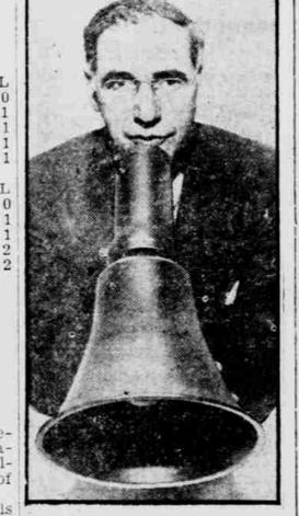
**MIGHTY MOUTHPIECE**—With the aid of tiny new electronic parts called "transistors," this newly-developed megaphone enlarges the human voice without external connections. Powered by small batteries the "transistors" do the work of vacuum tubes, eliminating the use of bulky high-voltage batteries and the need for an external power supply.
