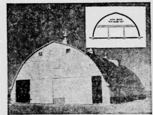
Strong Rilco Utility Rafters are factory fabricated from finish-grade, kiln-dried West Coast Douglas Fir laminations permanently bonded with waterproof resorcinol glue. They are delivered cut to exact lengths, drilled for connection hardware furnished, ready for rapid, labor-saving erection.
