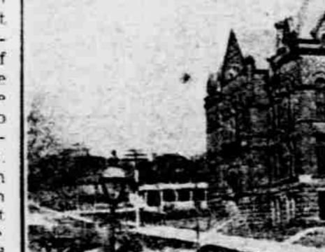
The above photograph of the Cass county courthouse was taken shortly after the turn of the century and used in an early day history of the county published years ago. The clock in the tower will soon be ringing out the hours again, thanks to hundreds of friends who have contributed their dollars to the Clock Fund.
