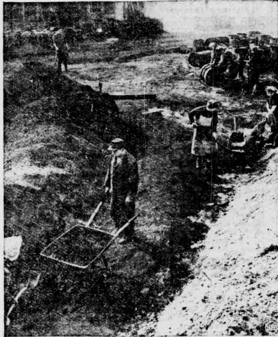
With real coal a scarce item in Berlin, "ersatz" (imitation) coal is being manufactured in the American sector. It's made of sawdust, coal dust and a tarlike substance, and has six times the heating value of the real thing. It's much cheaper, too. These men work between piles of coal dust and sawdust. (Photo by NEA-Acme staff correspondent Joe Schuppe.)
