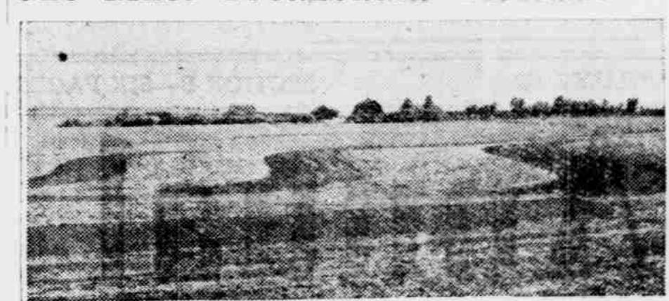
This picture shows newly-built terraces on a sloping field. They were built with a plow. They are broad-based and gentle-sloped so that they do not interfere with farming operations.—Photo by Soil Conservation Service.
