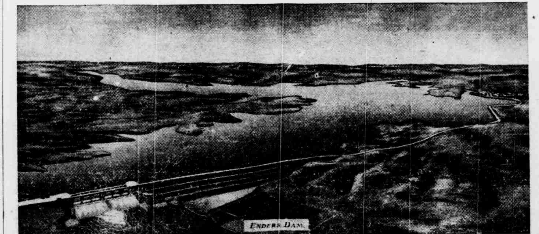
Designed to take the menace of the Republican river, which at times has caused millions of dollars in damage and taken scores of human lives, Enders Dam, as seen through an artist's eyes, will hold back the threatening flood waters to be used to irrigate the fertile soil from Enders, in Chase county, through Hays, Hitchcock, Red Willow and Furnas counties to the Harlan County Reservoir, below Orleans. Enders dam will be dedicated at a four-day celebration at McCook, starting May 29. Secretary of the Interior J. A. Krug will be among the important speakers appearing at the ceremony.
