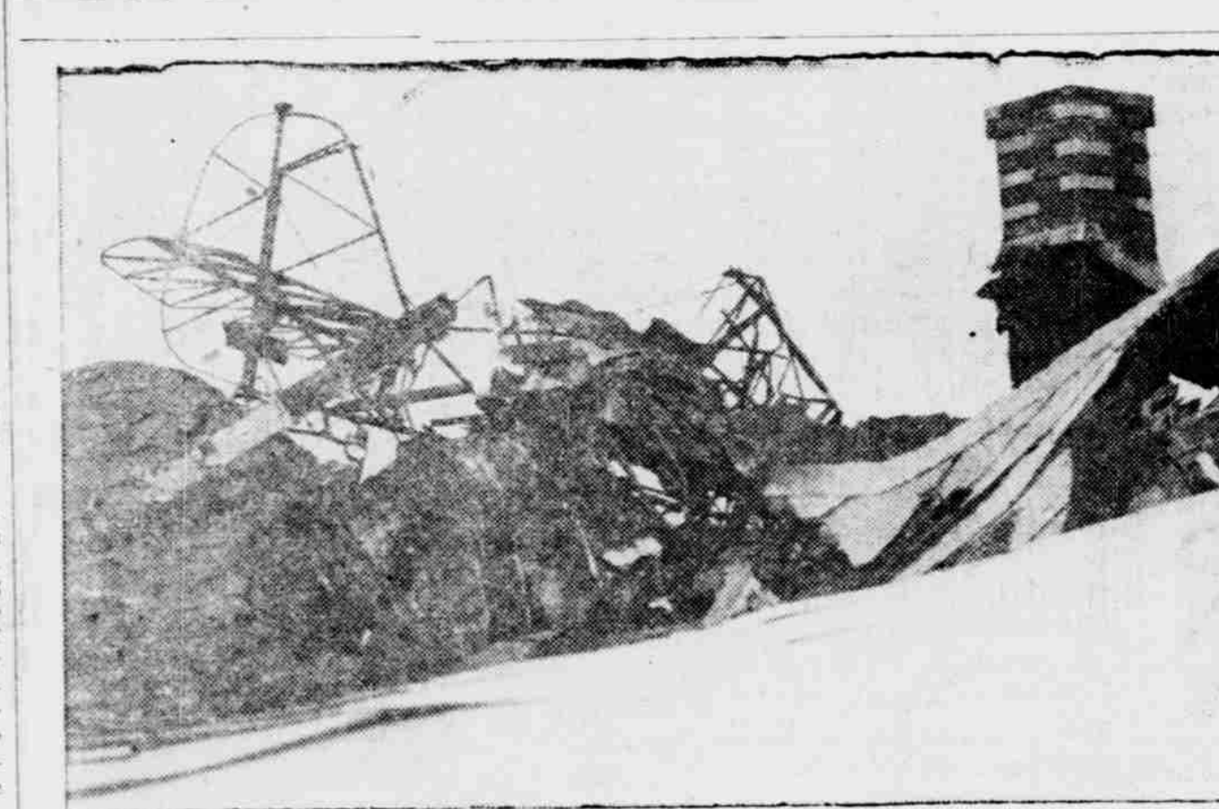
PLANE CRASHES INTO HOUSE—The metal framework of a light plane, its twisted, blackened remains, a grim reminder of a midnight frolic, protrudes from the roof of a Ft. Worth residence at 2541 Shirley St. The house was occupied by Mr. and Mrs. Samuel E. Hale, and all its occupants escaped without injury. The plane was piloted by Bobby T. Pirkle, 23, a Pacific-battle Veteran, who was enrolled at the Southwestern College of Aeronautics and who was killed in the crash. (NEA Telephoto)
