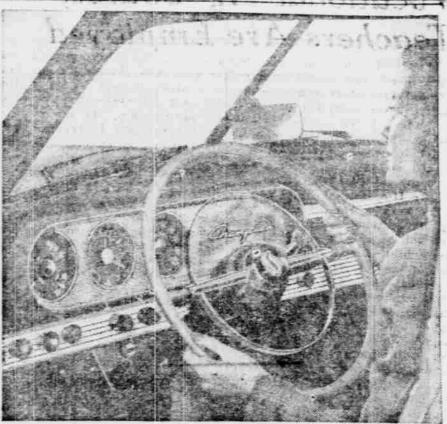
Aviation's cockpit influence can be recognized from this view the driver's compartment of the 1947 Studebaker Champion. Markings on the jumbo-sized dials are illuminated at night by nonglare "black light"-first developed for fighter planes during the war. Instruments are grouped for at-a-glance reading through the "maximum vision" steering wheel. Smart "airfoil trim" extends across the dash from the elliptical frame enclosing the instruments.
