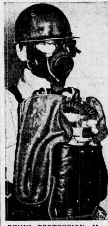
BIKINI PROTECTION-Members of navy salvage groups which will board "guinea pig" ships after the atom bomb is dropped in Bikini atoll lagoon will wear the lightweight plastic helmets and navy-tpye rescue breathing apparatus pictured
