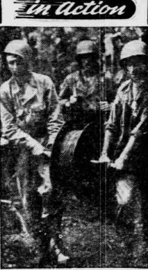
Signal Corps Photo Reeling out wire from an RL 31, in the steaming jungles of New Georgia-rain, insects and the
