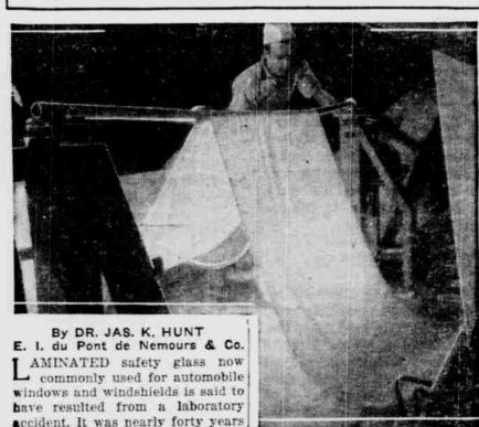
ago that a French chemist, Pro- Because of its great flexibility, lessor Benedictus, dropped a flask "Butacite" polyvinyl acetal plastic which had contained a solution of now used as the interlayer in nitrocellulose, a material made laminated safety glass can be rolled from cotton linters and used in up and shipped like a bolt of cloth. making quick-drying finishes. The =
