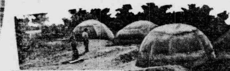
NEW PILL BOXES CONSTRUCTED HERE—New Haven, Conn.—Pill-Boxes constructed after a series of experiments will be inspected by officials of the War Department this week. 14 feet in diameter and 1 1/2 feet thick, the gun enclosures may be constructed in one day. They may also serve as bomb proof shelters.
