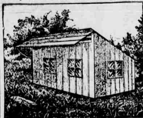
TURKEY HOUSE (FRONT VIEW). of Agriculture. In the front, near the top, is seen a ventilator, which should always be open except in exceptionally cold weather. The roosts are placed near the front of the house and are on the level. The back view shows the slide door, which should be left
