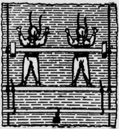
When it is impracticable for warships to go to dry dock for cleaning, divers work on staging to scrape the bottom.
