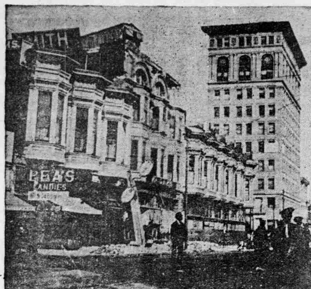
SKYSCRAPER THREE FEET OUT OF PLUMB.
