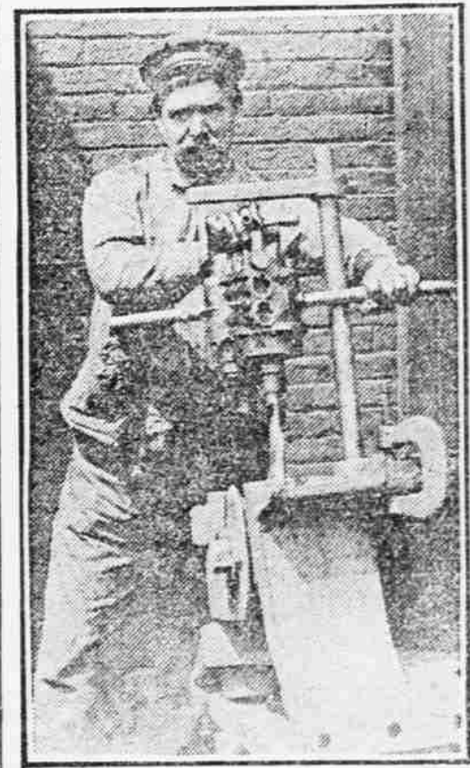
DRILLING A BATTLESHIP PLATE.
