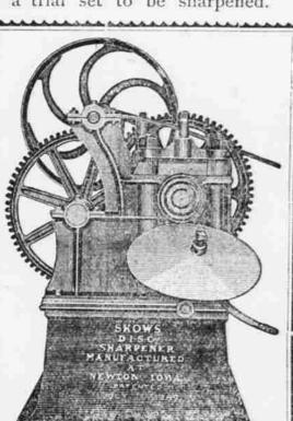
only 6 in Nebraska. Discs sharpened on this machine do better work and stay sharp twice as long as by the old hand method. The reason is that the disc is rolled instead of pounded, made from threeeighths to five-eighths of an inch larger, the steel is made harder and the disc naturally cut, easier, while the old method of pounding warps the disc out of shape and makes it rough.
