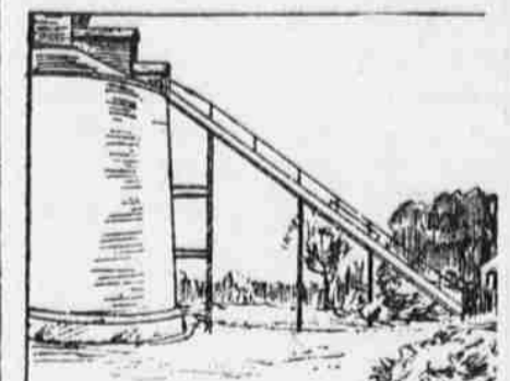
Filling With a Slat Elevator.
