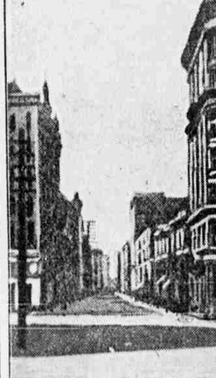
LOOKING UP MONTGOMERY STREET
