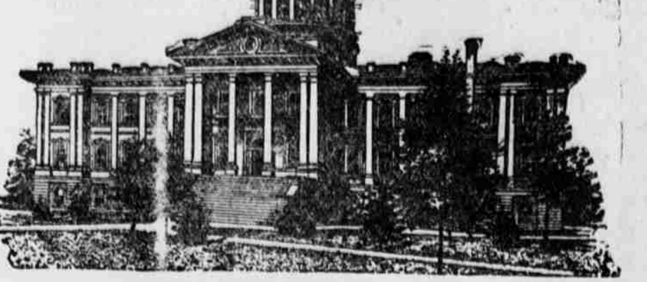
CAPITOL BUILDING, SALEM, OREGON. A Letter From the Executive Office of Oregon.
