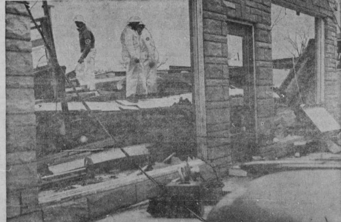
TYPICAL of some 1,000 civil defense volunteers are these rescue workers looking for survivors in suburban Standale's business district.
