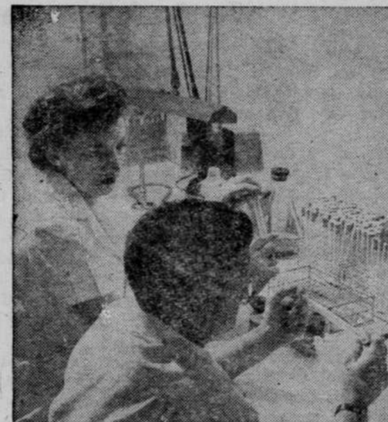
Animal tissue in tubes is inoculated with vaccine and let stand. If any live virus remains, it will multiply here, hence can be detected.
