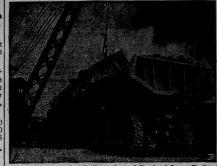
IRON SPRINGS, UTAH—A fleet of Fruehauf Dump Trailers, working in the huge Utah iron pits, is contributing nobly toward relief of the steel shortage in the West. Day after day these trailers, owned and operated by Utah Construction Company, deliver 750 tons of ore from the mine to the crusher at the railhead. Loads average 50 tons and each trailer makes 15 trips daily. Ore from the Utah mine is converted into iron the blast furnace of Kaiser Steel Mills, Fontana,
