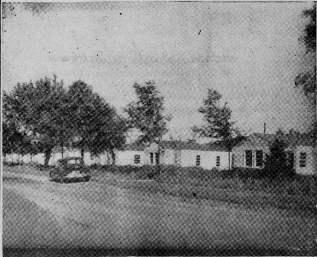
New Construction 83rd and Underwood
