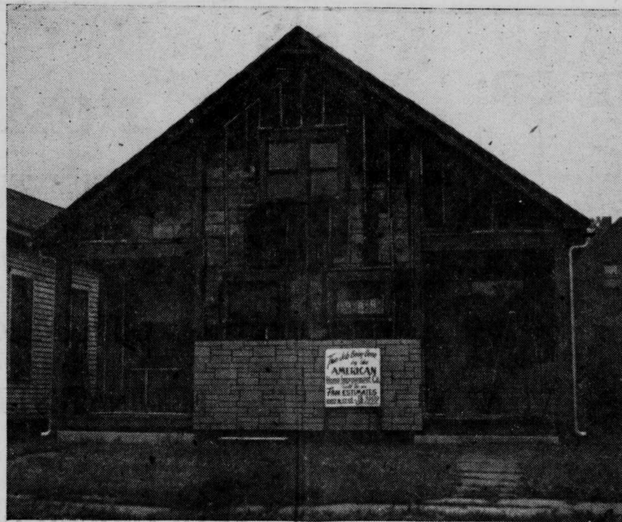
Unfinished Residence 2521 Ohio Street.
