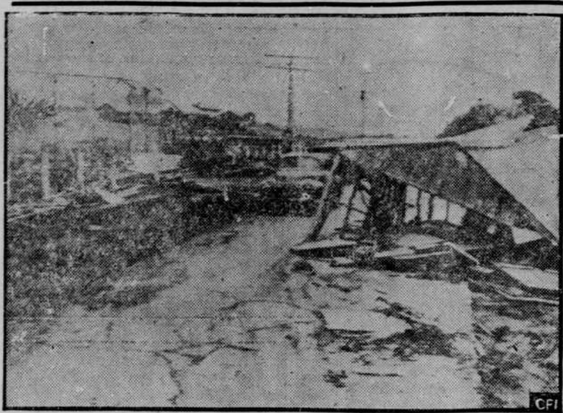
DAMAGE CAUSED BY TIDAL WAVE
