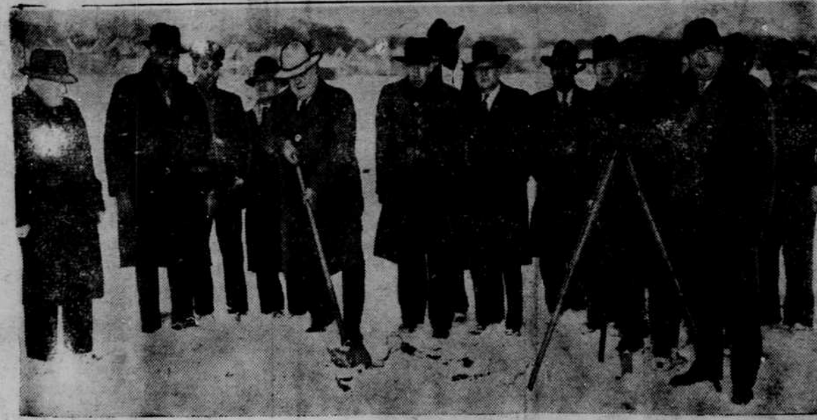
Left to right are William F. Scholman, plumbing contractor; Charles C. Gallaway, publisher of The Omaha Guide; Warren M. Alton, fireman; prospective home owner; Mr. Dee, Mayor Dan B. Butler; John Sutherland, excavation firm official; J. Dillard Crawford, another prospective owner; Ralph Ronau; Raymond R. Brown, secretary of the Urban League; the Rev. W. H. Phillips, president of the league, a workman; John Slavic, county clerk, holding surveying instruments, in front of workman.
