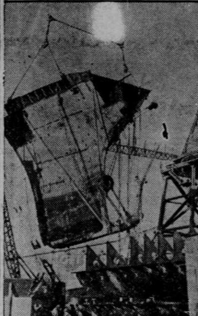
RICHMOND, CALIFORNIA — A new world's record for Liberty ships of four days and fifteen and one half hours from keel laying to launching was chalked up at the shipyards here when the epic-making vessel, the "Robert E. Peary" slid down the ways.
