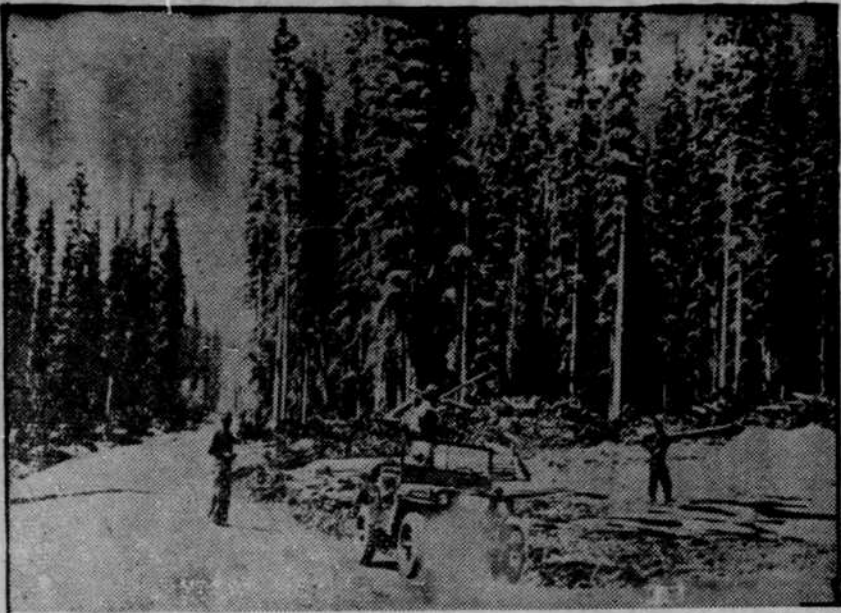
NORTHERN CANADA—Soundphoto—A portion of the International highway, from the United States to Alaska, being completed through virgin forests. It will make a military road protected by a chain of coastal mountains from the Northwestern United States to our Alaskan defense area, through the Dominion of Canada.
