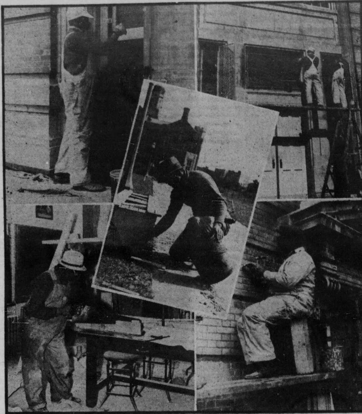
WPA Workmen Repair School Buildings Throughout the Nation As Schools Open
